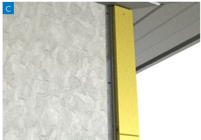
Double Flange Sealant Backer flanking stacked Corners
